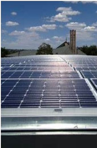
Solar panels overlooking Sacred Heart Catholic Church.
